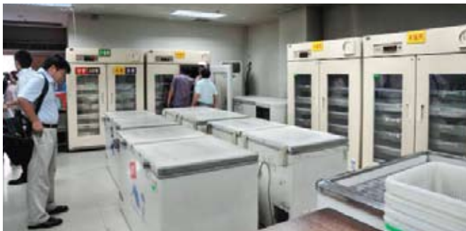
The Blood Storage and Control room which stores and controls the supply of blood as well as filling orders.
